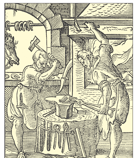
Figure 18 Late medieval illustration showing smiths at work. Note the waist-level hearth in the background and the anvil set in a wooden block.
