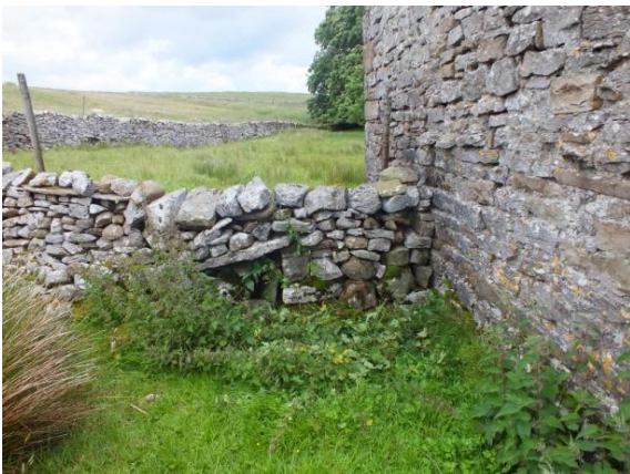
Fig. 9.25 Nettles masking a collapsed creep running from field to field (Phil Carroll)
