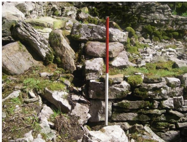
Fig. 15.6 The straight joint indicating the doorway from bodystead to parlour (David Johnson)
