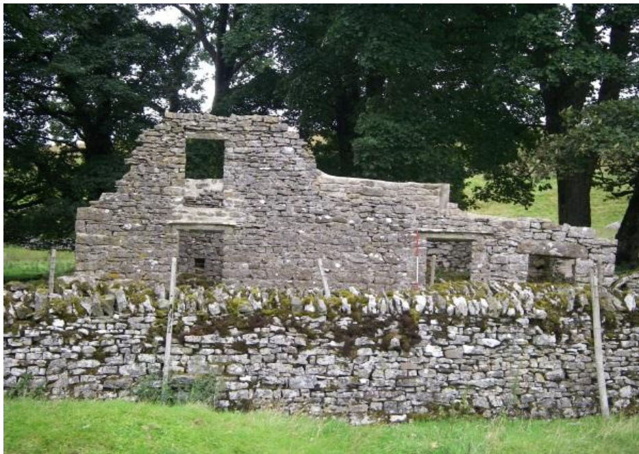
Fig. 16.6 The house frontage after consolidation in August 2017 (David Johnson)
