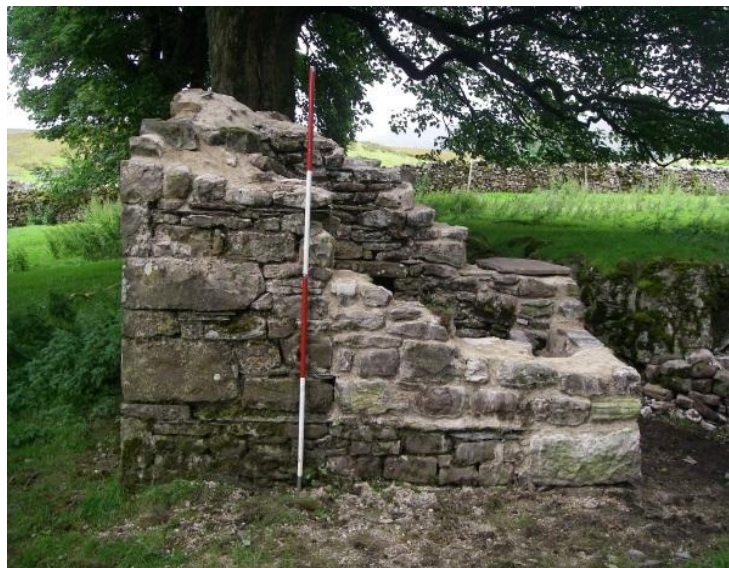
Fig. 16.4 The privy – the 'out-office' in contemporary parlance – on completion of consolidation works (David Johnson)
