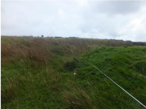
Fig. 9.22 Wall – what wall? The case of a disappearing wall (Wall no. 12) (Phil Carroll)
