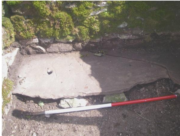
Fig. 15.7 The seat or shelf in the porch. The floor level lies below the later accumulation of soil (David Johnson)
