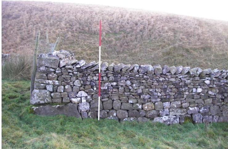
Fig. 10.48 Thorns 12, north-east corner (David Johnson)
