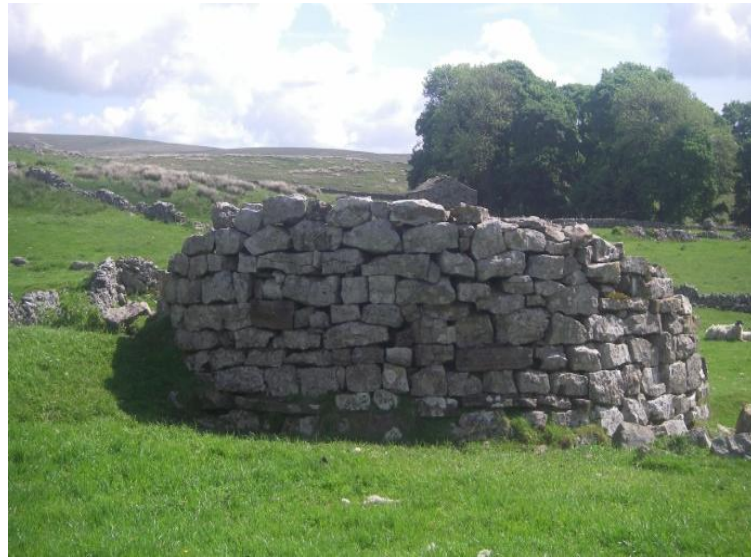
Fig. 16.7 The lime kiln after stabilisation works (David Johnson)
