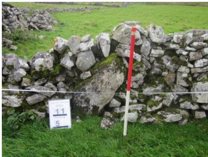
Fig. 9.10 Wall no. 11, displaying the characteristics of older walls (Pat Carroll)
