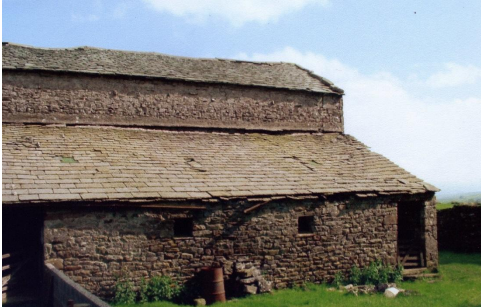
Fig. 10.43 Thorns 10, north elevation and outshut in 2004 (Frank and Muriel Laver)
