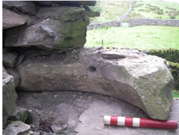
Fig. 15.3 The fire window lintel as found reused in the front face of the house. The view here is on the inside of the wall where it had been hidden from view prior to building consolidation works (200mm scale) (David Johnson)
