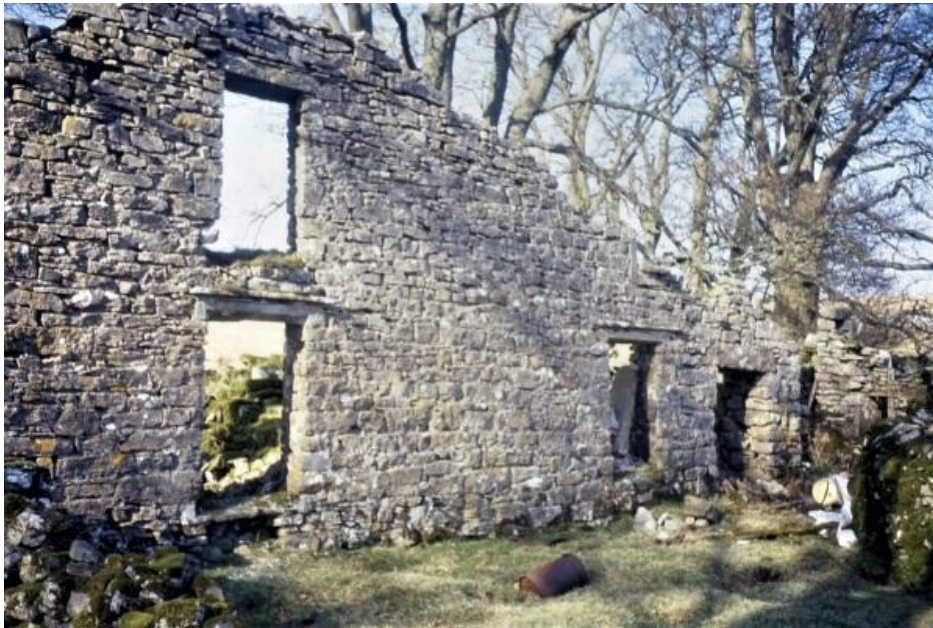
Fig.16.5 The house frontage in 2003 (David Johnson)
