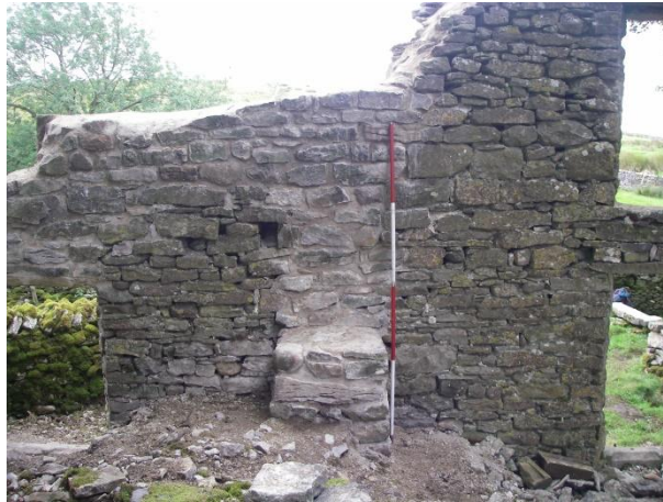
Fig. 15.5 The restored stub from the second-phase dividing wall between bodystead (to the left) and parlour (to the right) (David Johnson)
