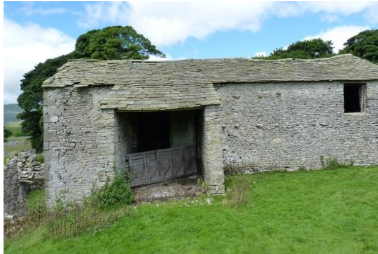
Fig. 10.61 Thorns 10, bank barn, in 2016 (Dianne Wall)
