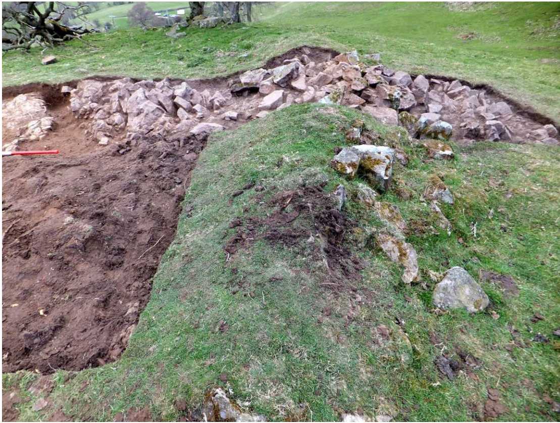
Figure 27: Circular 19C. enclosure dry-stone wall foundation.
