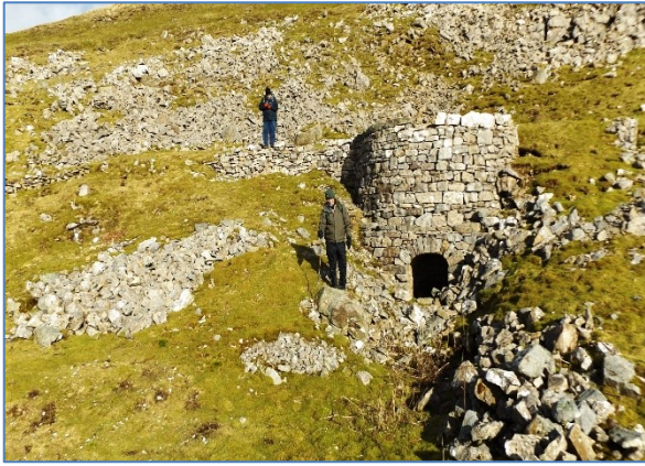
Figure: 27 lime kiln at Winterings Pasture and access roadway above for loading the kiln [W13]
