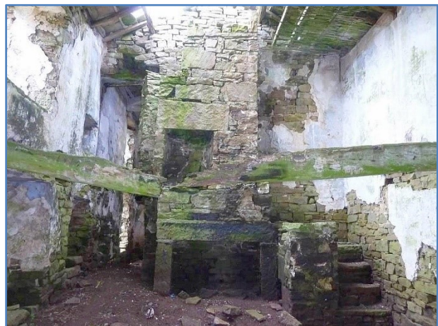
Figure: 113 Brownsey House © Stephen Eastmead
