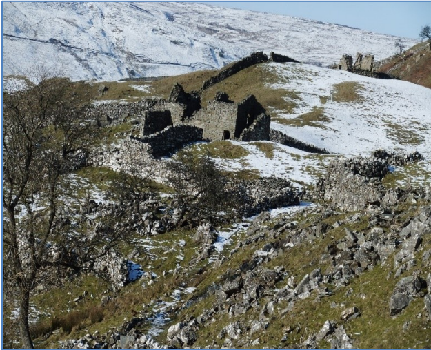
Figure: 24 Ruined farmstead near Hugill House
