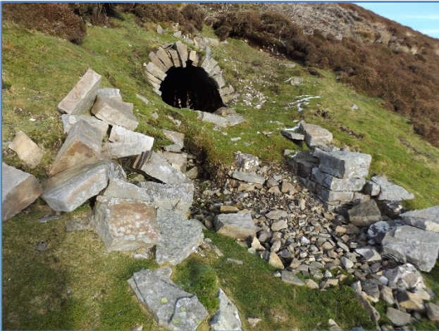
Figure: 110 The portal to the Brownsey Level
