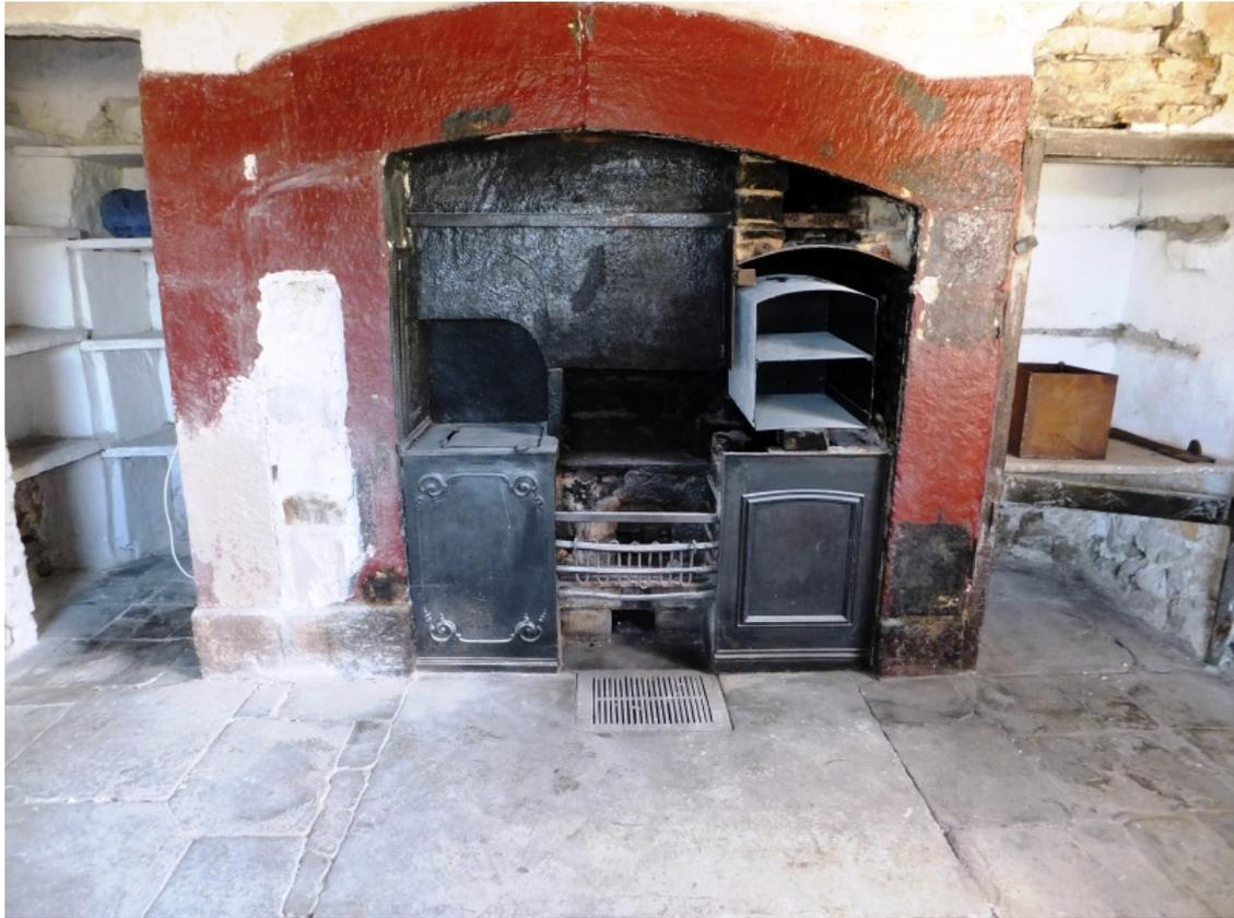
**Figure 2: The C19<sup>th</sup> range and ash pit grate in the west room**
