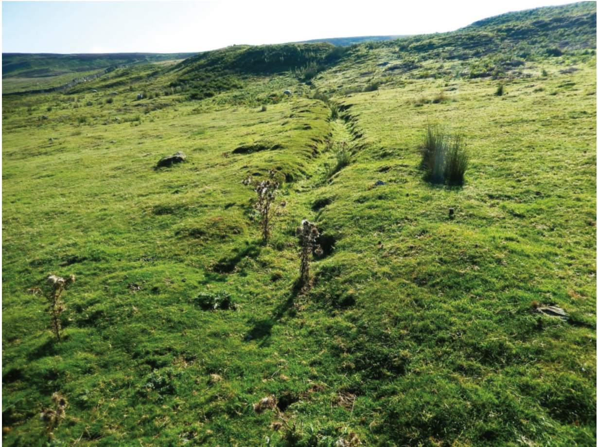
Looking from the south-east corner of Juniper Gill Plantation at the leat that connects the moorland reservoir with Juniper Gill.
